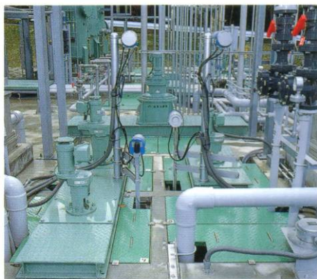
●凝集沈殿槽
