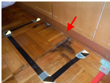
2-1 床板の腐朽
